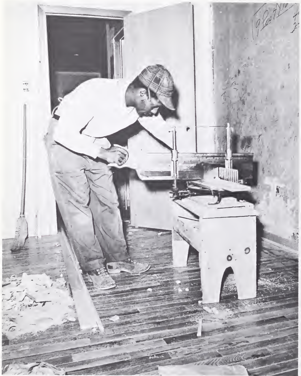
CHIP REHABILITATION IS EFFECTED BY LOCAL COMMUNITY CONTRACTORS
